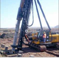
Hydraulic piling rigs with hydraulic or diesel impact hammers are mainly used for driving precast concrete piles but in some cases also for sheet piles, beams and pipe piles.
