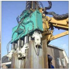
Our hydraulic sheet pile press mounted to an ABI Mobilram is often the only solution in case of soft ground conditions and when no vibration at all is allowed due to nearby delicate structures or underground utilities.
