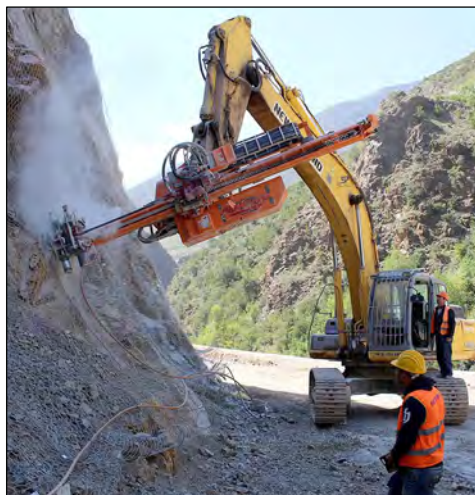
ADD-ON DRILL MAST For anchors, micropiles and blast holes
