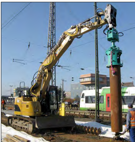
ADD-ON AUGER DRIVES Pre-drilling hard soil and much more
